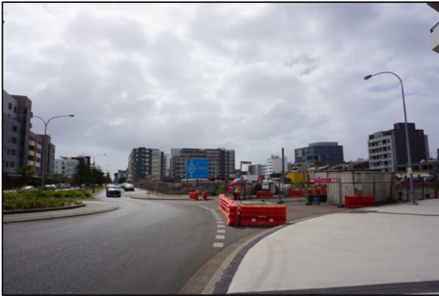
FIGURE 12: VIEW EAST, CONTEXT OF SITE 1 LOCATION, VIEW EAST DOWN HONEYSUCKLE DRIVE, WORTH PLACE VISIBLE CURVING TO RIGHT OF PHOTO. SITE 1 IS LOWER AREA OF LAND IN CENTRE OF IMAGE SURROUNDED BY MESH FENCING ETC (SOURCE: CURIO 2018)
