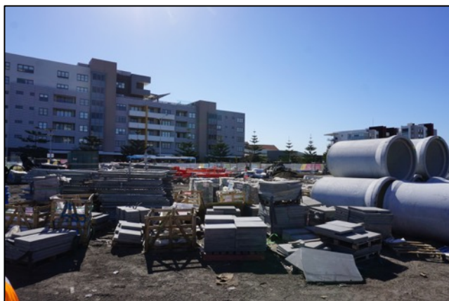
FIGURE 35: SU2, VIEW EAST ACROSS CONSTRUCTION MATERIALS STOCKPILE (SOURCE: CURIO 2018)
