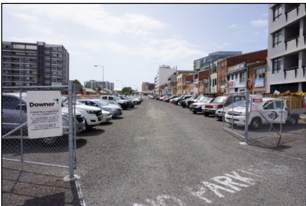
FIGURE 16: VIEW EAST ALONG FORMER RAIL CORRIDOR (SOUTHERN PART OF SITE 2), CURRENTLY USED AS PARKING/CONSTRUCTION STAGING FOR CONSTRUCTION OF LIGHT RAIL (SOURCE: CURIO 2018)
