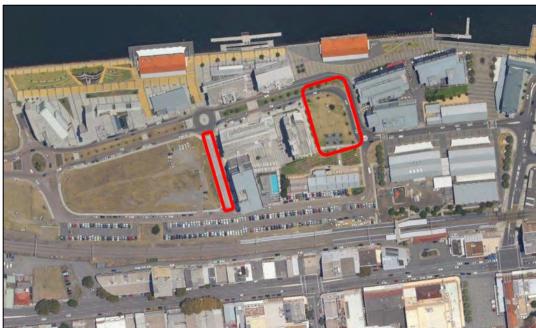
FIGURE 7: 2012 AMAC STUDY AREA WITH REFERENCE TO SITE 1, 2 AND 3 LOCATION (SOURCE: AMAC 2012: 8)
