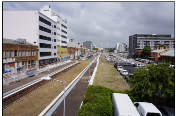
FIGURE 29: VIEW FROM CIVIC STATION, WEST TOWARDS SITES 2 AND 3 (VISIBLE AS CARPARKS IN BACKGROUND) WITH SITE 1 FURTHER IN THE RIGHT BACKGROUND OF IMAGE (SOURCE: CURIO 2018)
