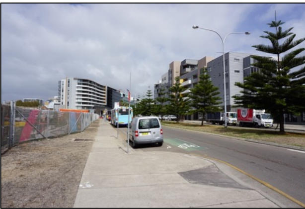
FIGURE 26: VIEW WEST ALONG HONEYSUCKLE DRIVE, SITE 1 VISIBLE IN LEFT (SOURCE: CURIO 2018)
